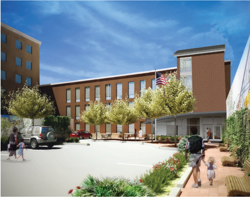
The Impact Services Veterans and Family Housing Center will provide 26 units of housing in the Kensington section of Philadelphia. Rendering by Kramer+Marks Architects.
